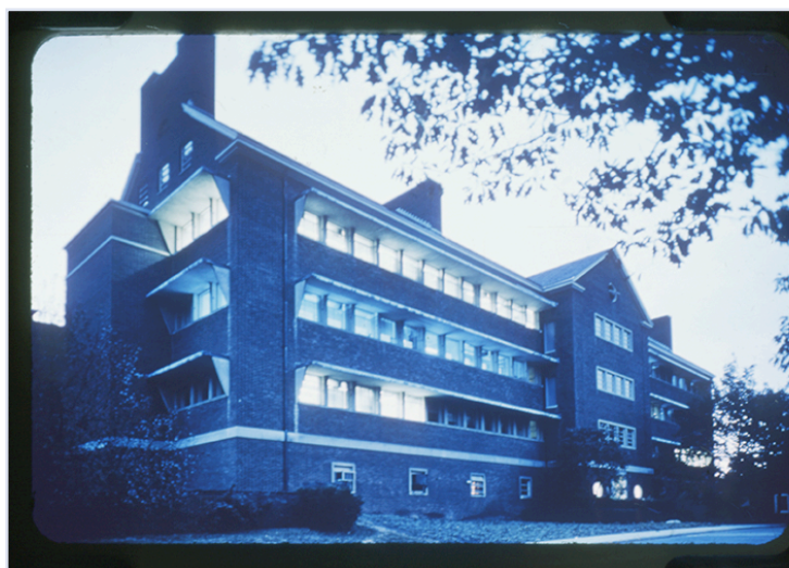
NIH’s Building 7, on the Bethesda campus, boasted a state-of-the-art biosafety system when it opened in 1947: superheated grids sterilized air as it passed through the ventilation system; labs had ultraviolet lights that were turned on each night to sterilize surfaces; access to the laboratories was through decontamination locks; and concrete window canopies instead of fabric shades (that might become contaminated). Above: At night, the building “glows” with ultraviolet light.
